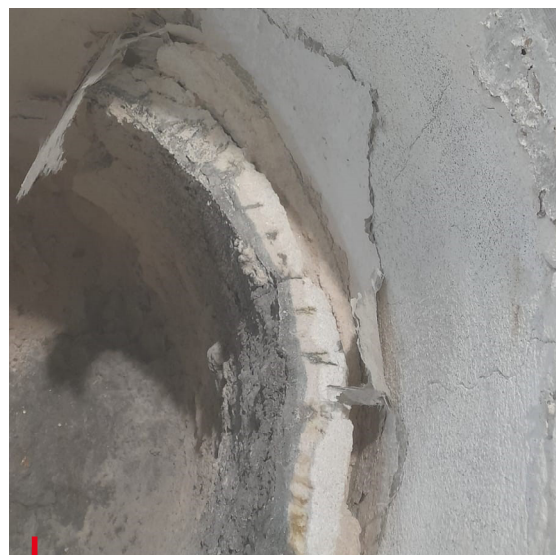
Higher powder thickness at the back of lining
